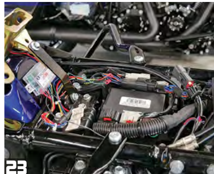
22 Next, Tony finds a good place to attach the ground wire to the frame (arrow).
